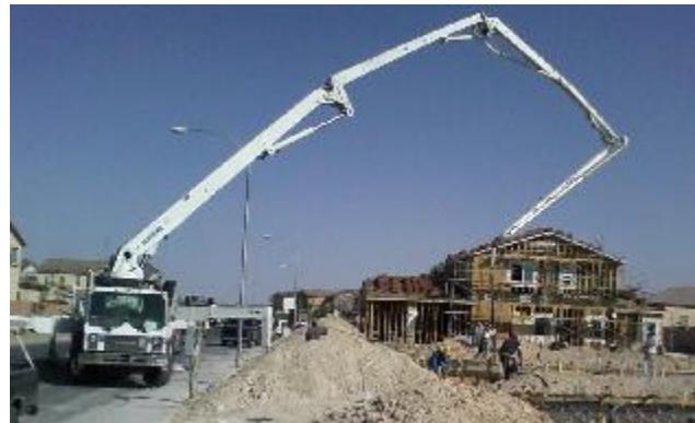
Figure 11: Grout Delivery Truck and Pump (image provided by all-concrete-cement.com)
